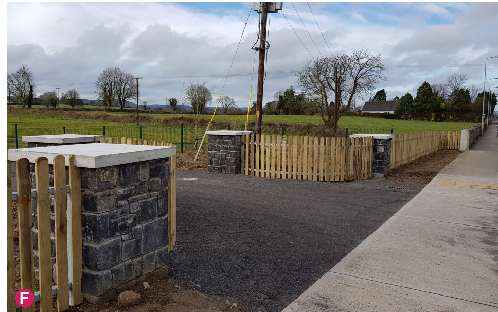
Figure 24. New entrance to Town Park from Newcastle West Road (R522)
