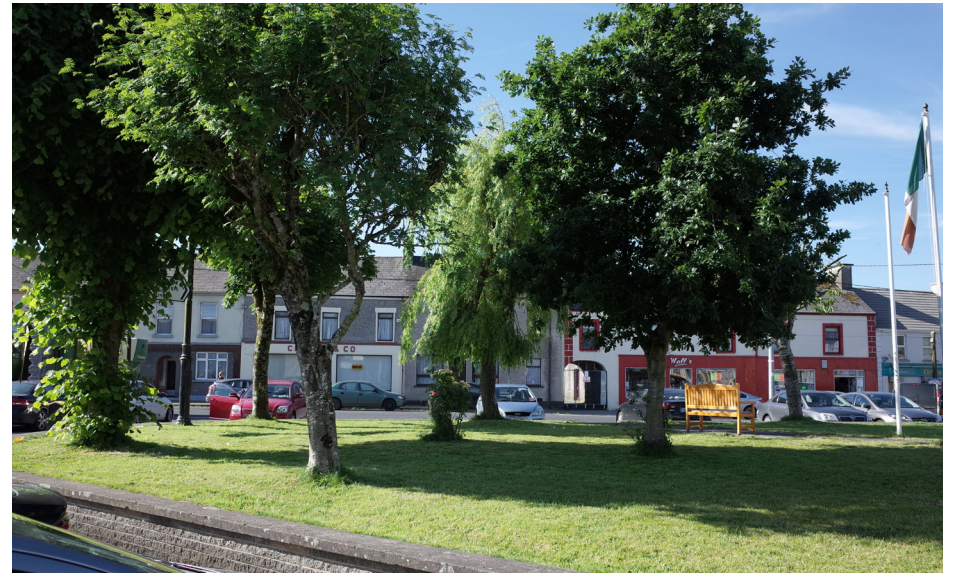
Inappropriate landscaping within the central garden. There are too many trees for the size of the green area and some of the species are not suitable for this location.
