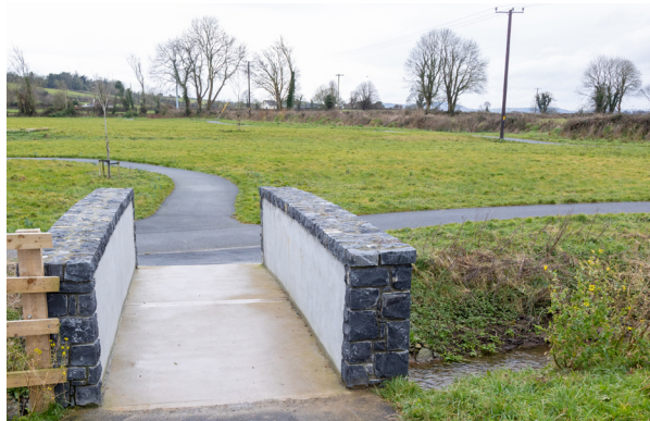
Recently installed Lower Bridge
