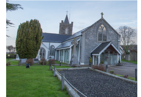
St Bartholomew's Church
