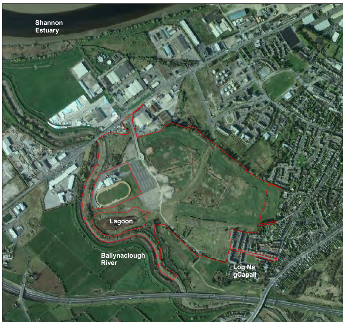
Figure 2.1 Aerial photograph indicating the extent of the masterplan area
