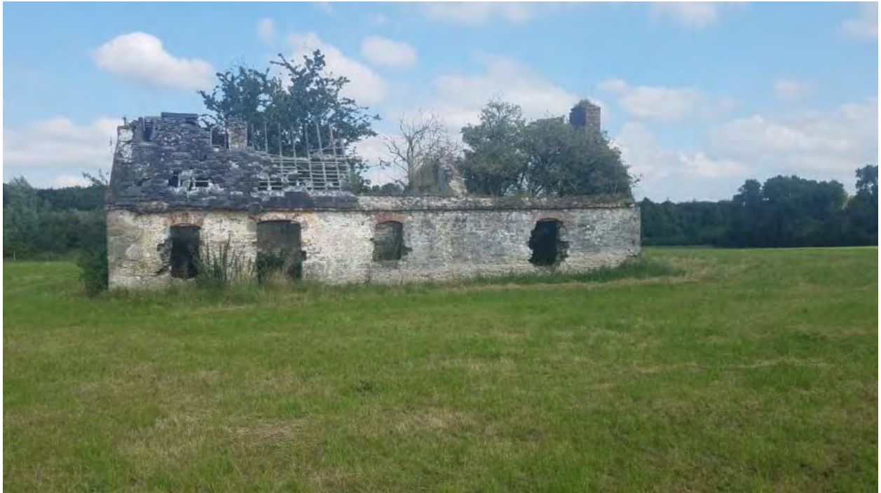
Image 9: Abandoned house in middle of site 1
