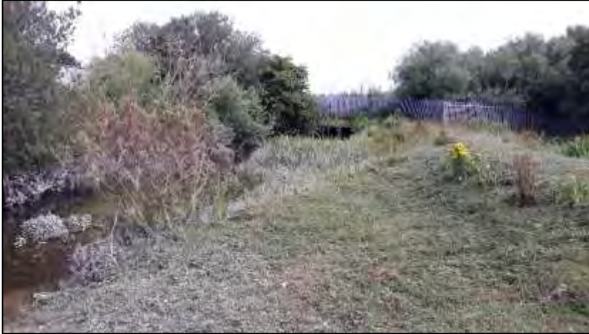
Photo 18: Location F – Railway crossing (Structure 3965) facing upstream
