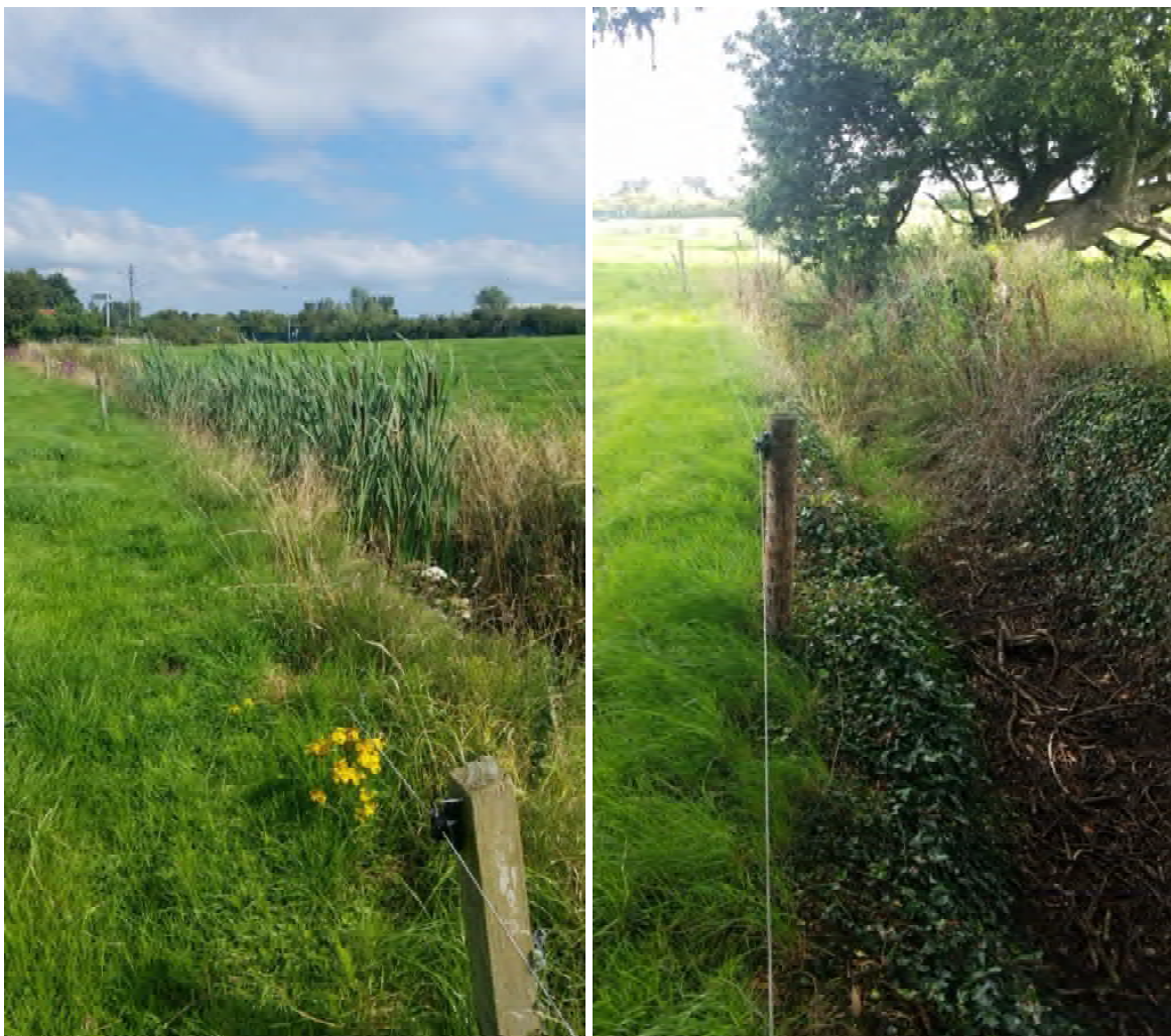
Image 6: Existing OPW channel crossing southern boundary of Site 2 (east)
