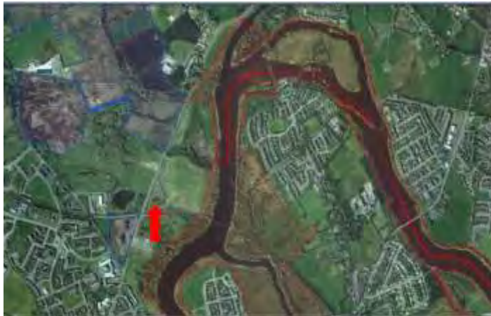
Figure 1.8: The red arrow shows the compensatory habitats for works on the Limerick main drainage scheme in the early 2000s. It is a series of constructed wetlands and wetland vegetation.
