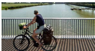
Example of cycle - pedestrian bridge at rail bridge
