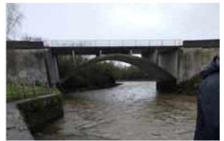
Slipway and view to the bridge (N69)
