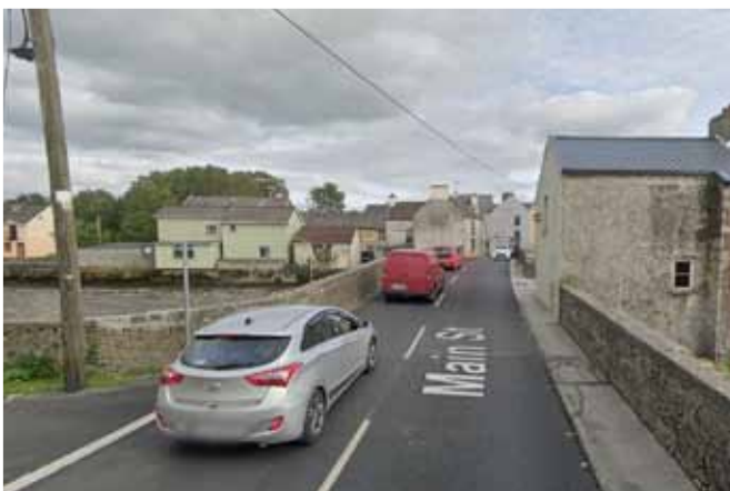
Main Street at the bridge (from west)
