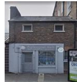
35 Mallow Street – RPS 3106
