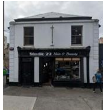
29 Mallow Street - RPS 3103
