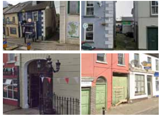
Existing pedestrian lanes and coach house entrances. Derelict properties can offer opportunities for off-street infrastructure.
