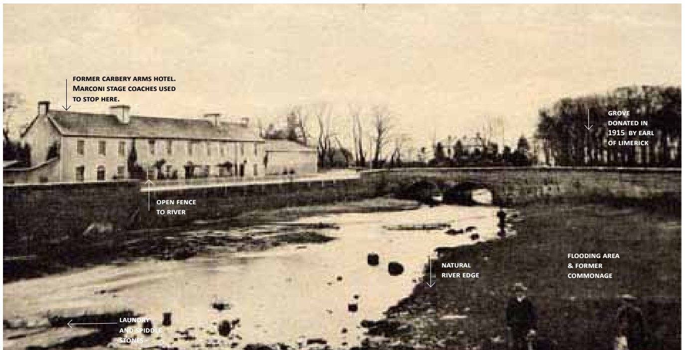
Figure no. 43: Historical image of Morning Star River Park
