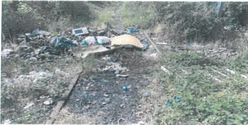
Image above shows unlawful waste disposal along the trackside verge adjacent to Garyglass Avenue
