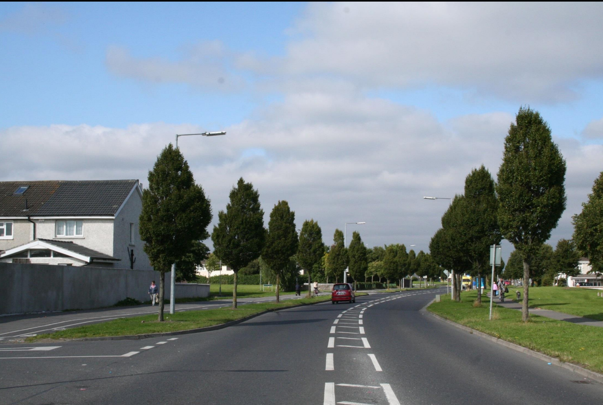
Neilstown Road, Dublin
