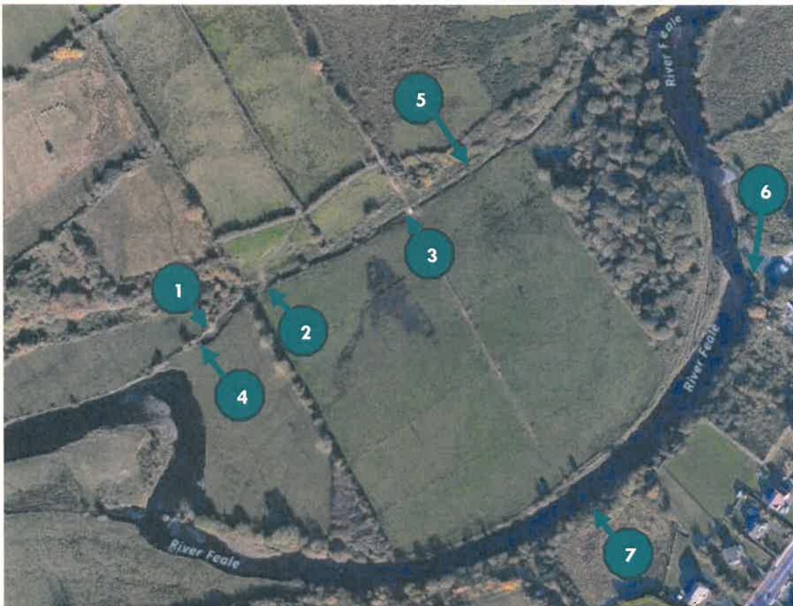
Figure 3.5: (1) Proposed Sheet Pile Weir site, (2) Former river crossing (A), (3) Former river crossing (B), (4) Breach channel, (5) Catchment Channel, (6) Existing intake, (7) River Feale Meander
