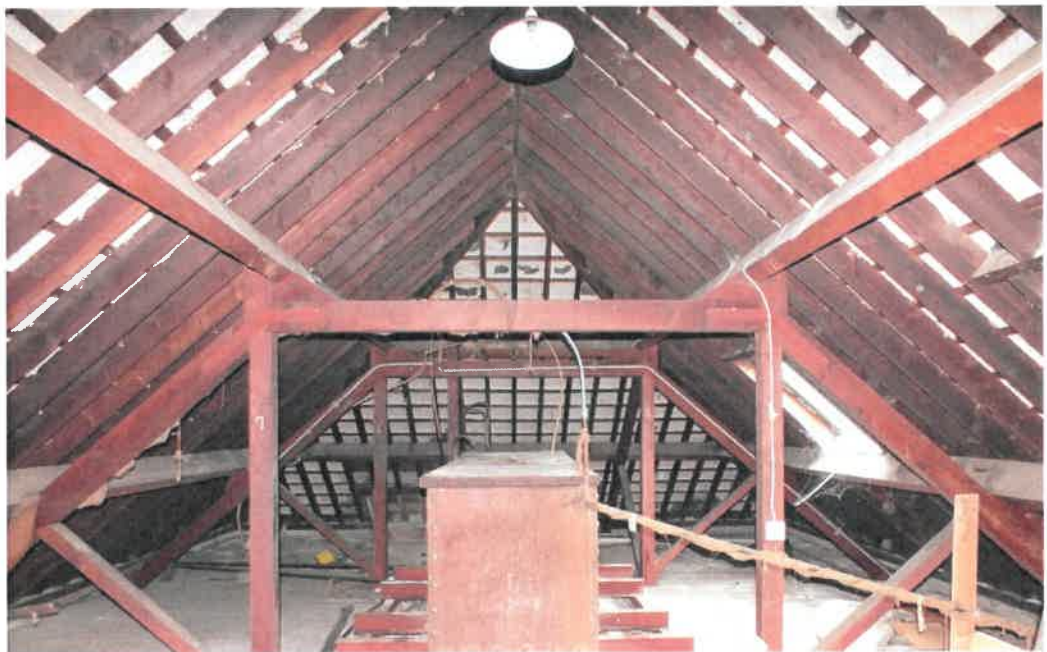
Plate 2020/A(5): An example of the excellent roofing structures that characterise the construction techniques used throughout the various building phases of the Convent Complex's evolution from its foundation through to the completion of the Chapel in the 1950s. Note the white lime plaster beneath the slates. Known as parging, it provided a seal against drafts through the natural slate cover but was also breathable- allowing accumulated moisture in the building to evaporate through.
