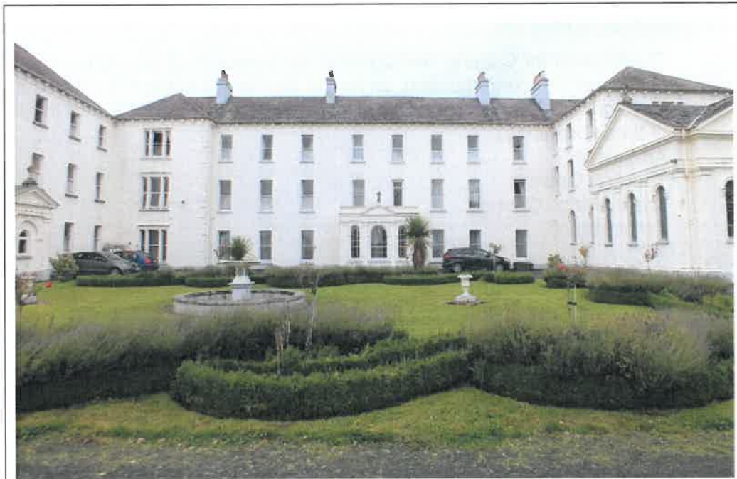
Plate. 2020/A(1): View, taken from the south showing the irregular layout of the complex and the haphazard fenestration patterns evident in the elevations. The Chapel is visible to the righthandside of the image and is identifiable from the Romanesque arches on the windows.
