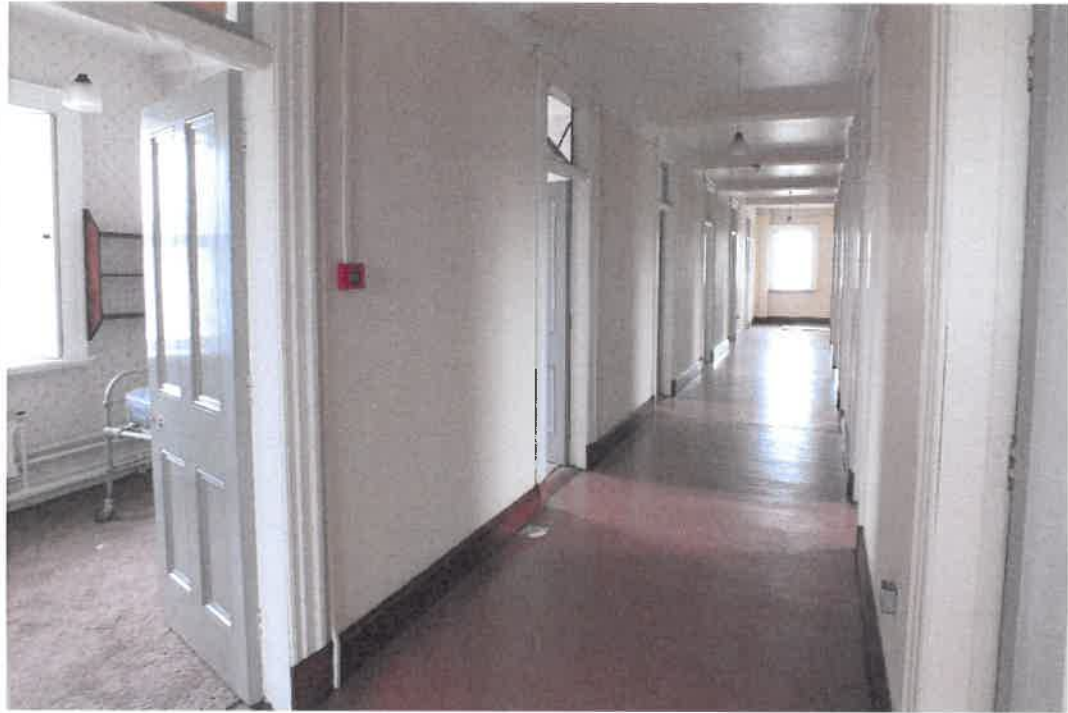
Plate 2020/A(4): One of the many corridors on the second and third floors, off which the individual rooms that provided sleeping accommodation for the members of the Order of Mercy's Community in Doon over many decades.
