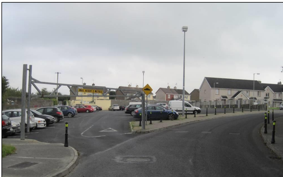
Figure 6.1 Council owned car park to the south of Main Street
