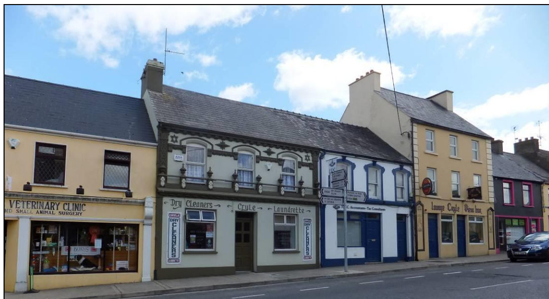
Figure 2.5 Examples of Protected Structures, Church Street, Abbeyfeale
