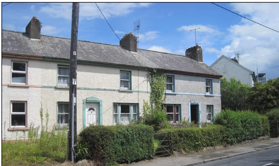
Figure 10.2 Vacant units at Colbert Terrace
