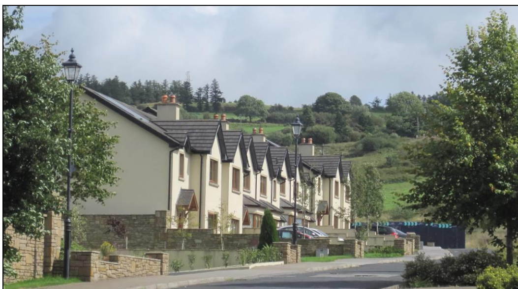
Figure 4.1 Completed units in Ellis Wood Housing Estate
