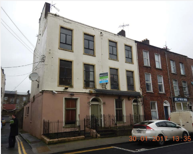
Catherine Street - Works from the Derelict Sites Inspection Team
