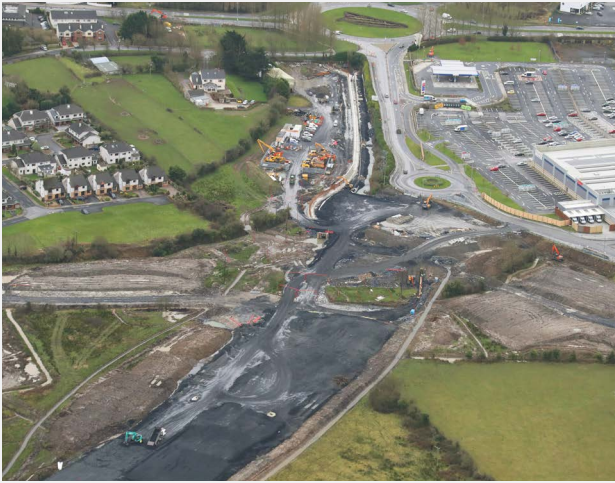
Coonagh Knockalisheen Distributor Road Phase 1 Under Construction
