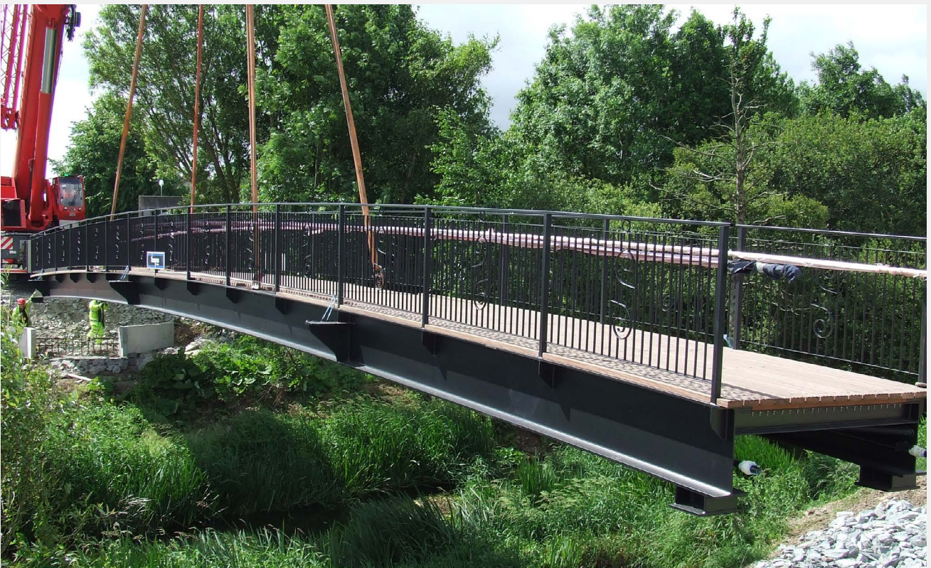
New Footbridge opened in Kilmallock.
