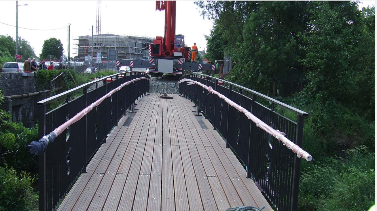
New Footbridge opened in Kilmallock.
