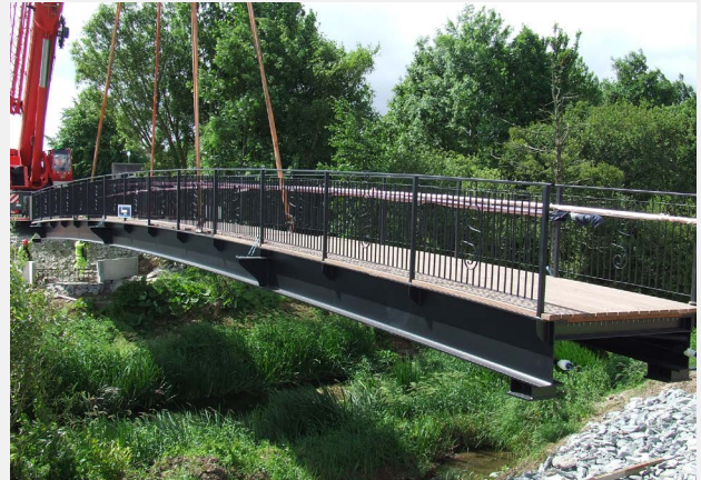
Cappamore-Kilmallock Installation Of Kilmallock Footbridge
