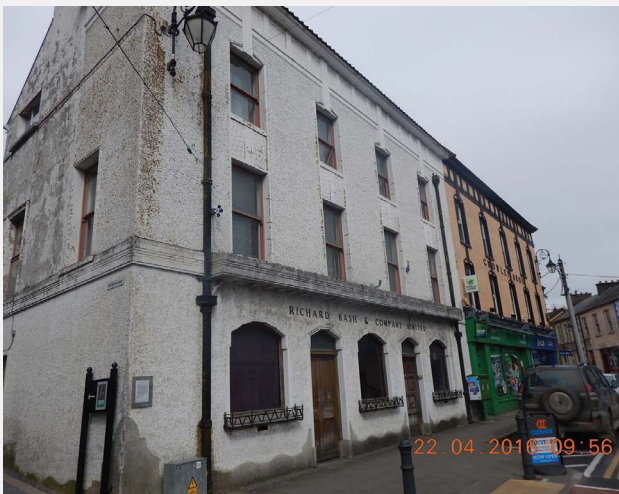
The Square, Newcastle West - Works from the Derelict Sites Inspection Team
