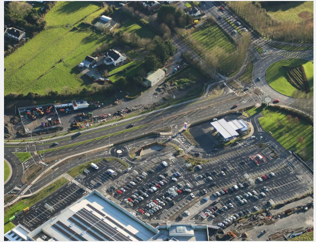
Coonagh Knockalisheen Distributor Road Phase 1 Complete
