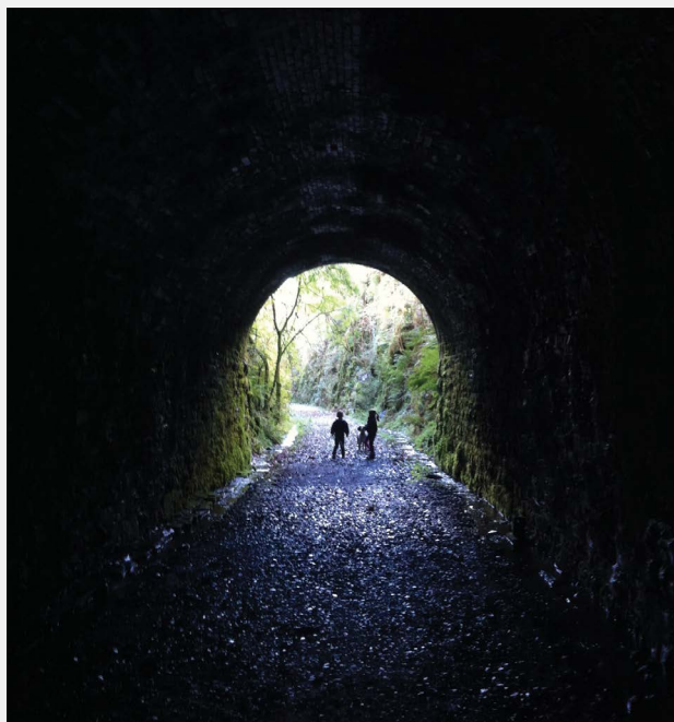
Barnagh Tunnel on the Great Southern Greenway
