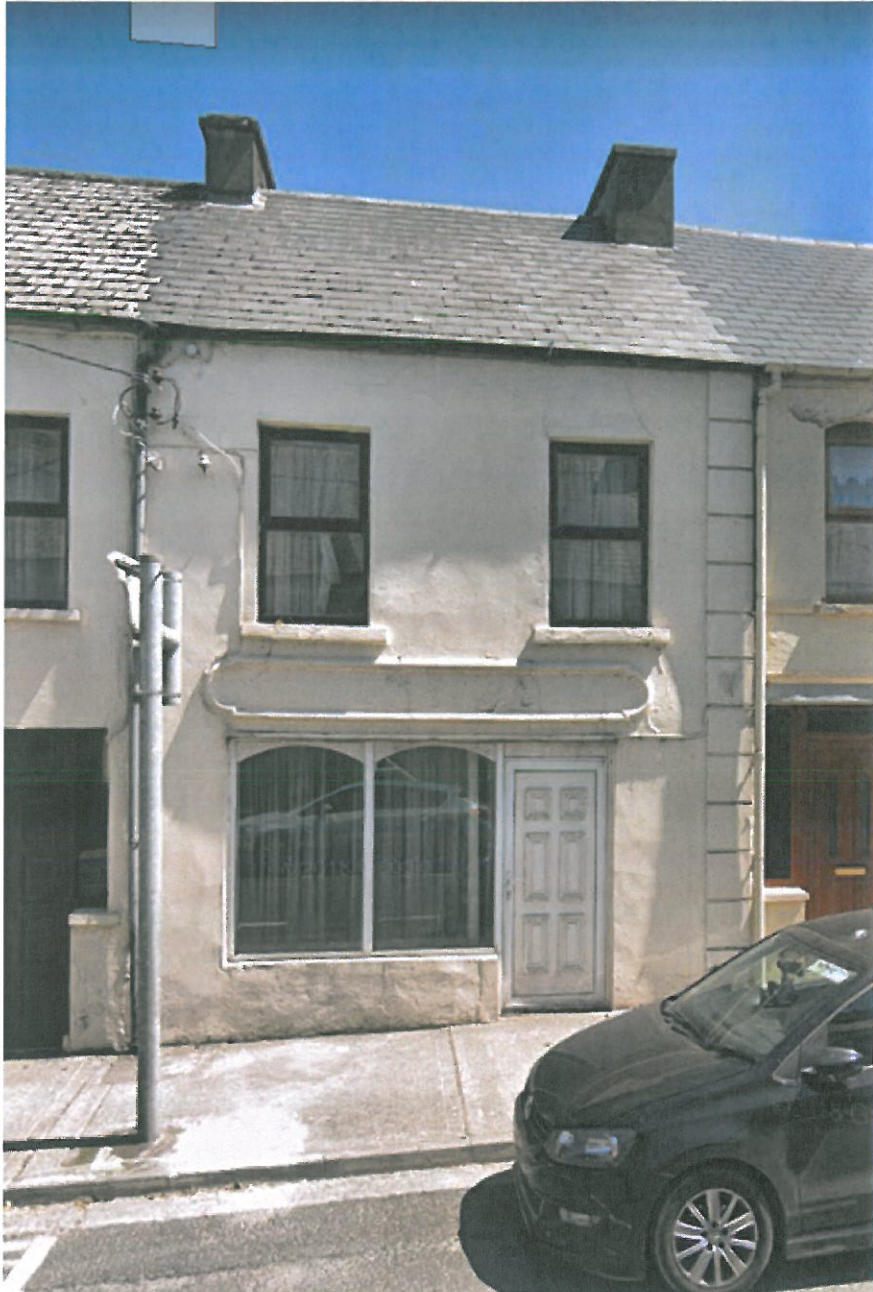
Houses to be refurbished
