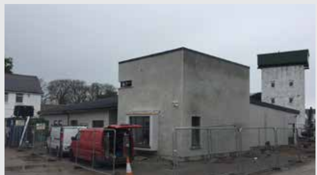
Construction underway at Cuan Mhuire, Bruree
