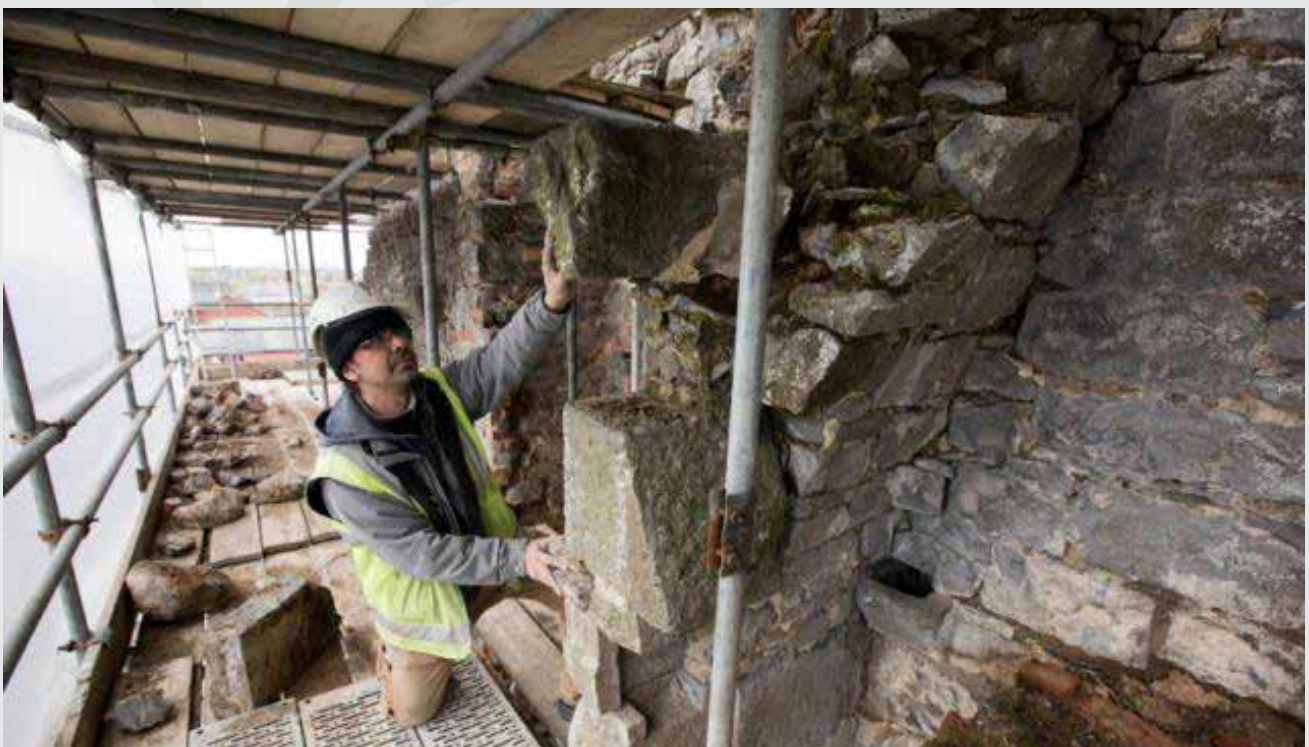
An expert stonemason working on the Fireplace Site during Phase 1 Stabilisation Works in 2017
