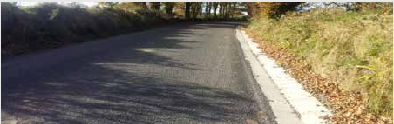
Severe weather fund – concrete channel on L1516 Ballintober
