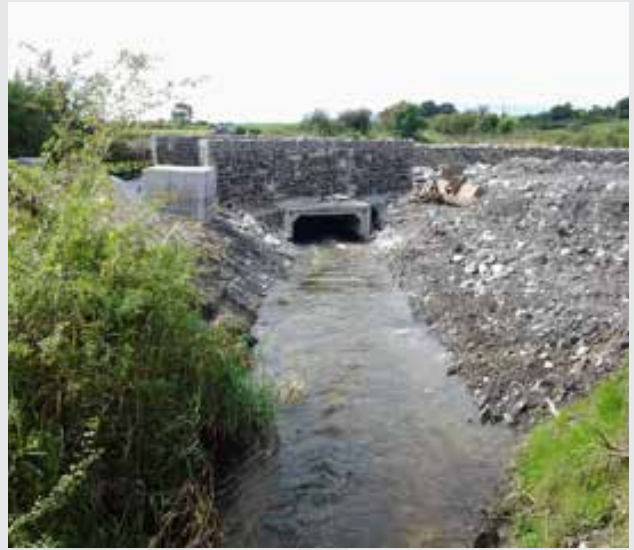
Bridge refurbishment at Courtbrown, Rathkeale.
