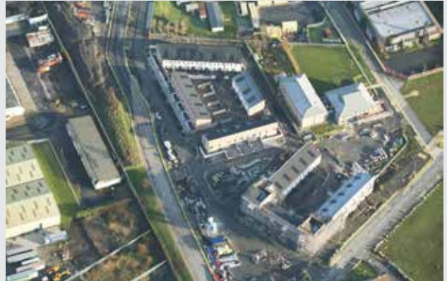
Churchfield Phase 1, will complete in early 2018 providing 42 new housing units
