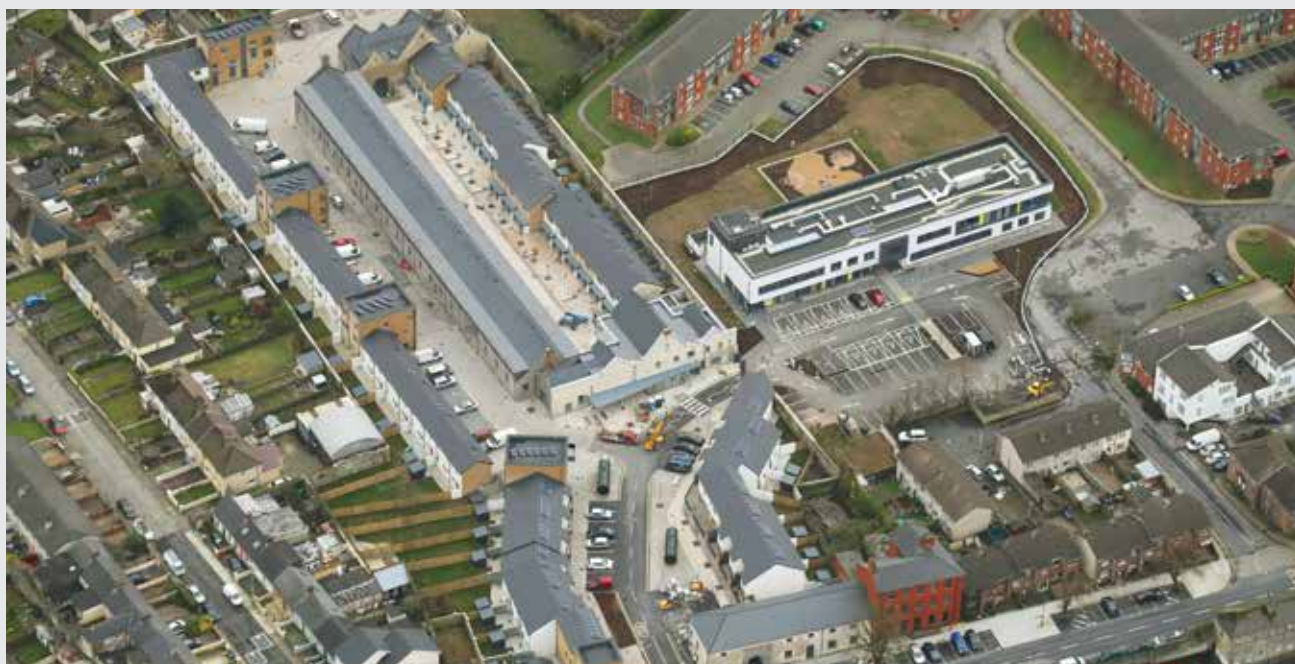
An aerial view of the new Housing Development at Lord Edward St., 81 units have been allocated in this development.
