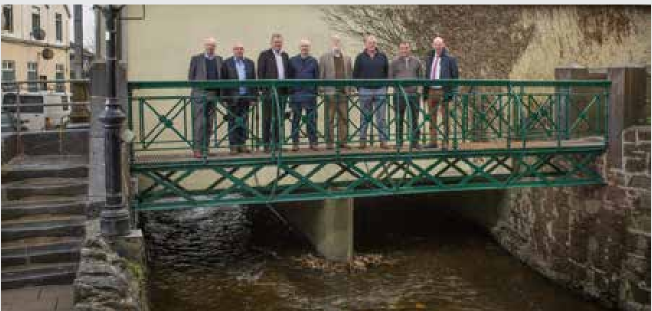
Curlings Bridge, Newcastle West
