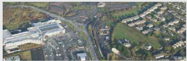
Construction of the Coonagh-Knackalisheen Road
