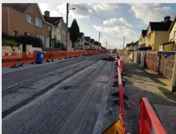
Roadworks in Progress at Flood Street, Garryowen, Limerick. Works carried out by Roadstone. Plane out entire existing concrete pavement. Replace with Asphalt surfacing
