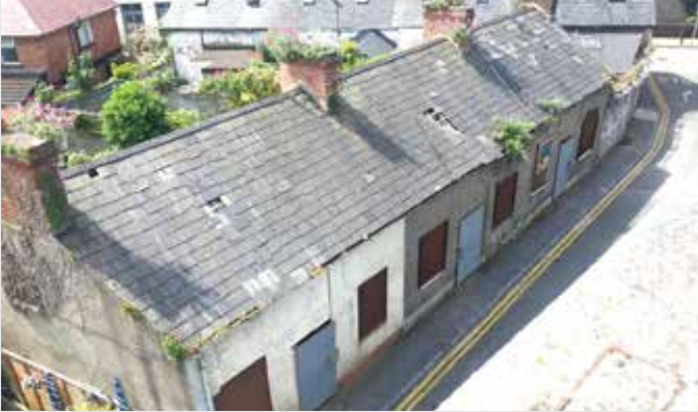
The major refurbishment of 8-10 Gaol
