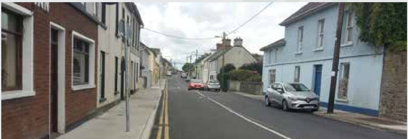
Completed works at Bridge Street Cappamore.
