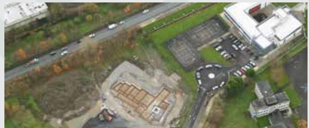
Child and Family Centre under construction in Southside Education Campus
