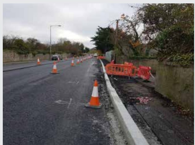
Roadworks in Progress at Annacotty, Limerick. On-going works on R445 at Annacotty. The scheme cost €600,000. The works were undertaken by Roadstone Ltd and was carried out during November and December 2017 during night-time. This scheme had a positive impact on traffic entering and leaving Limerick City during peak periods reducing queuing lengths.
