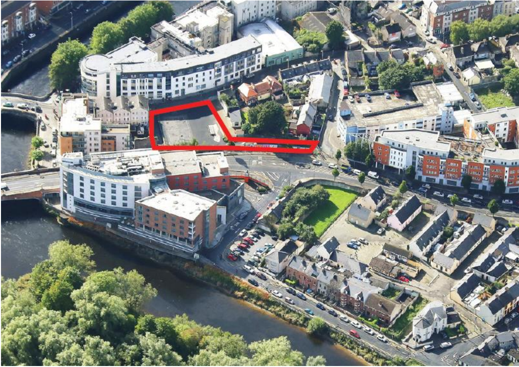
Figure 1: Annotated aerial view of site with LCCC lands shown in red
