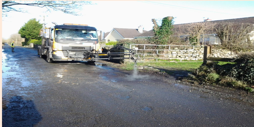
Tar Patching Askeaton
