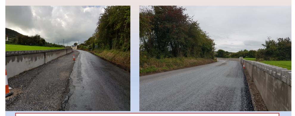
Photos 3 & 4 - Shows the ongoing strengthening works in front of the wall at Nicker and completed works on 18th September 2017. The works completed at Nicker include surface water drainage, public lighting ducting, road reconstruction and double surface dressing. The placement of the public lighting poles is outstanding.
