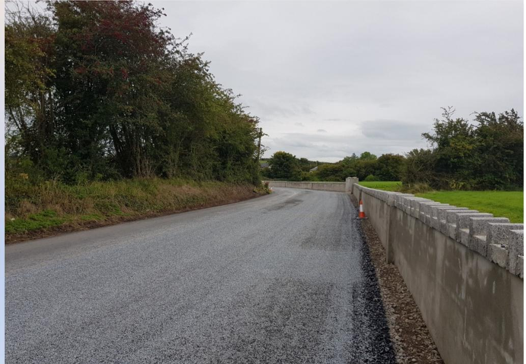
Photos 3 & 4 - Shows the ongoing strengthening works in front of the wall at Nicker and completed works on 18th September 2017. The works completed at Nicker include surface water drainage, public lighting ducting, road reconstruction and double surface dressing. The placement of the public lighting poles is outstanding.
