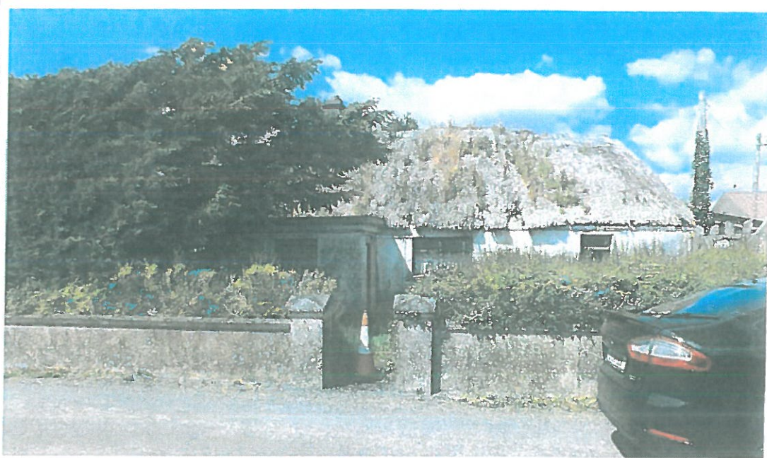
Plate B1: View of the principle (southern) elevation of Flynn's Thatched House from the roadside. Masked by the overgrown trees forming a hedgerow, the areas to the west of the porch have collapsed, while much of the remainder of the roofing cover has become invaded by plant growth.
