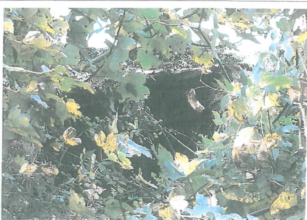
Plate A2: Close up view of the collapsed area encircled in Plate A1.
