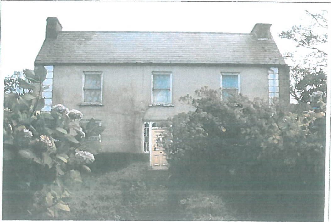
Plate C1: View of the principle (northern) elevation of O'Connor's Farmhouse, dating to November 2000. Apart from the timberwork, the only painted elements are the stucco quoins, which are not in line with the building's returns.
