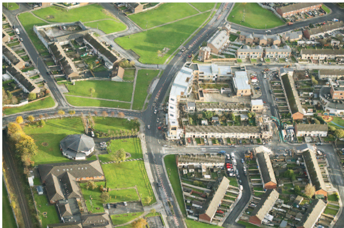
Cliona Park Phase 2 site which will deliver 10 housing units, image taken in January 2017
