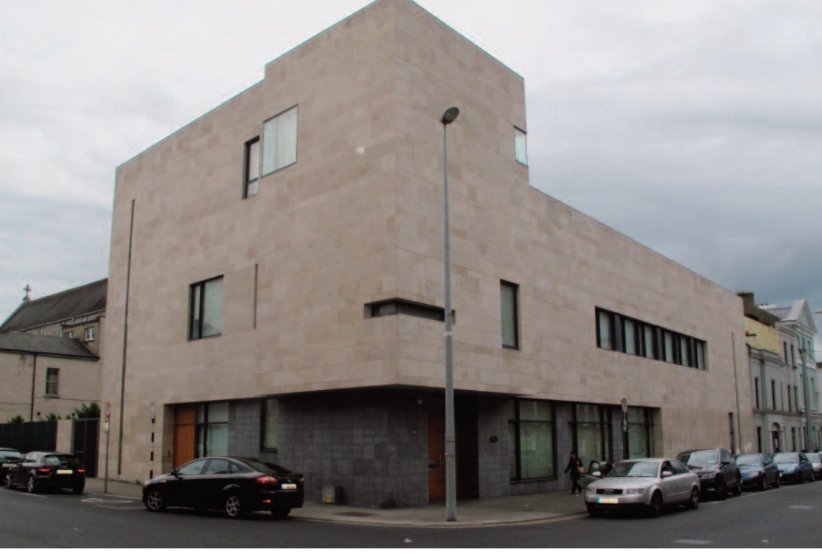
The former Biblical Centre, Cecil Street, which will be repurposed as the Production & Digital Skills Academy
