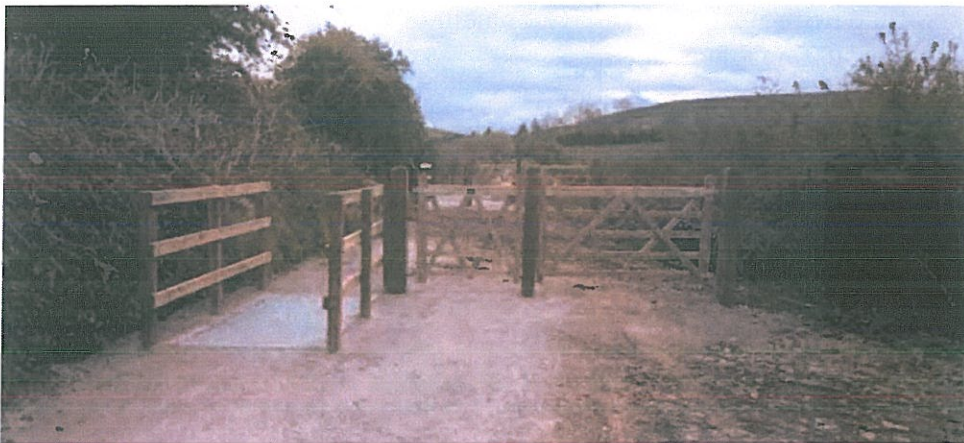
Proposed new gate system – Cattle grid and fencing will allow passage of cyclist and pedestrians separately
