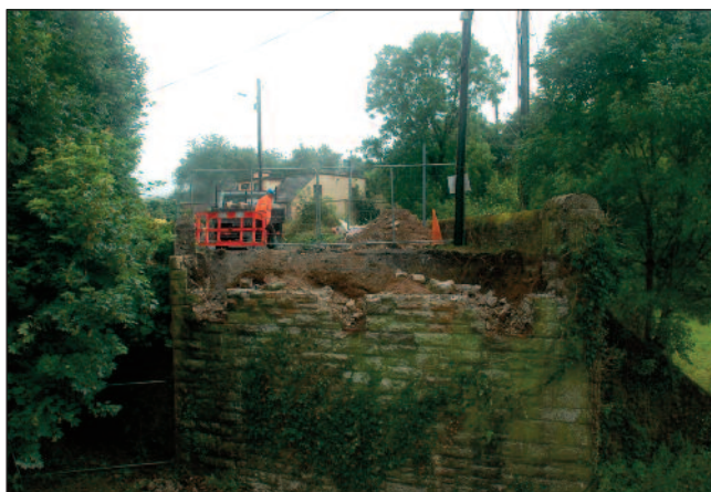
Glasha Bridge – old deck has just been dismantled and removed.
