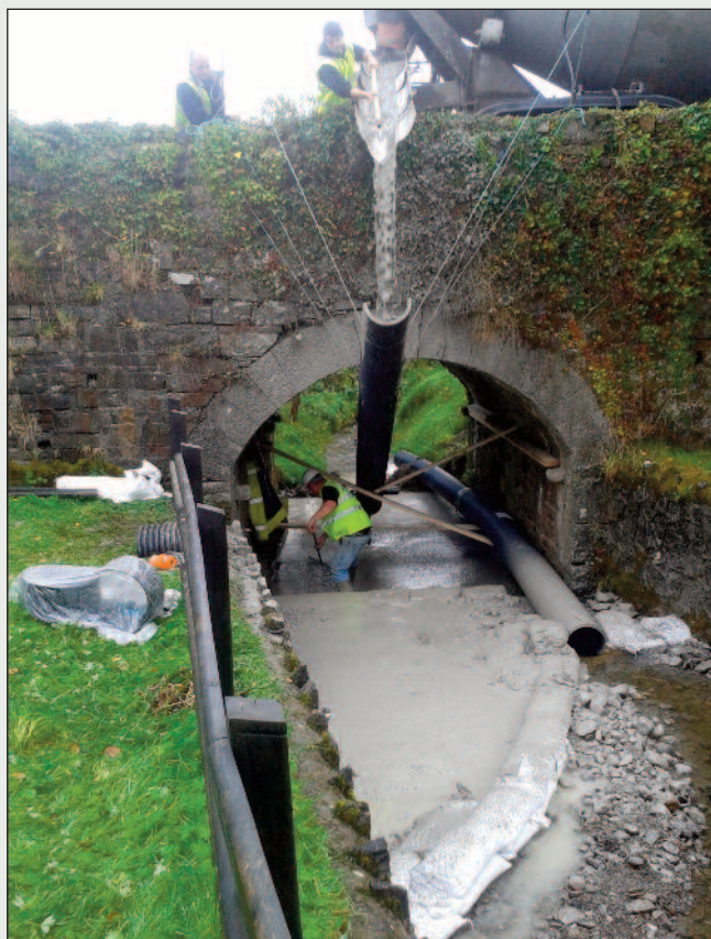
Strand Bridge – underpinning/floor being poured
