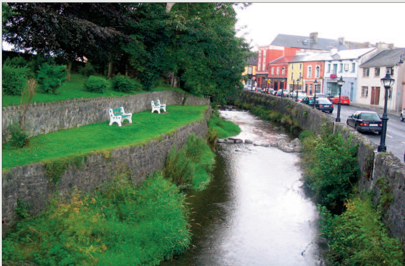
River Arra at North Quay, Newcastle West
