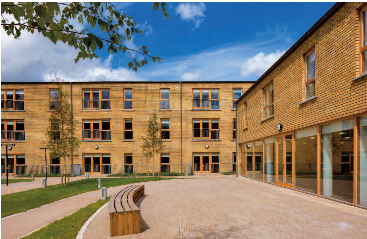
Vizes Court, Joseph's Street - 29 Units Completed in July 2014
