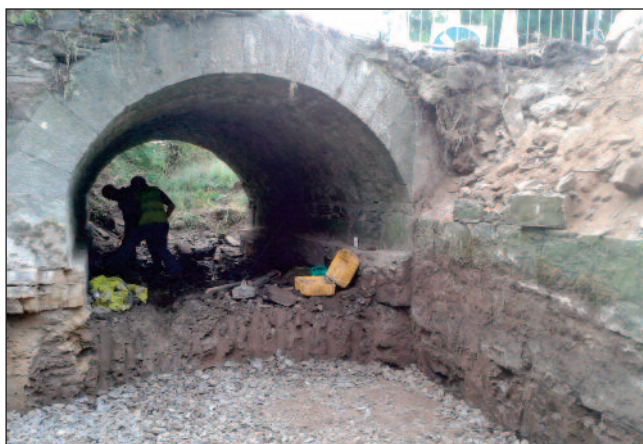
Coon Bridge – Base has been prepared for bridge extension.
