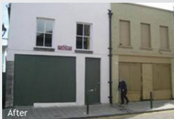
Nicholas Street refurbishment - After.
