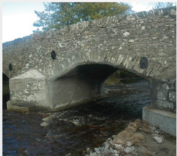
Loghill Bridge L6106.
