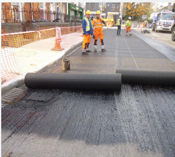
Road Resurfacing works on Newenham Street..
