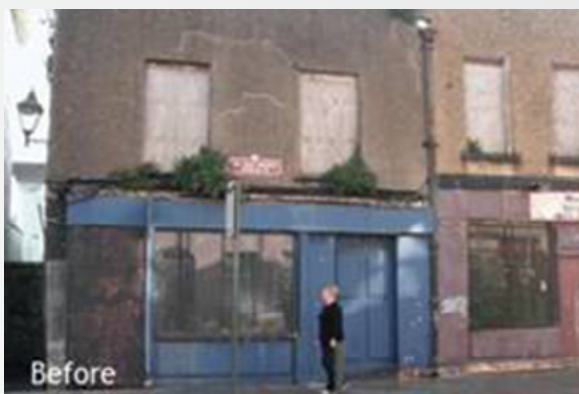
Nicholas Street refurbishment - Before.
