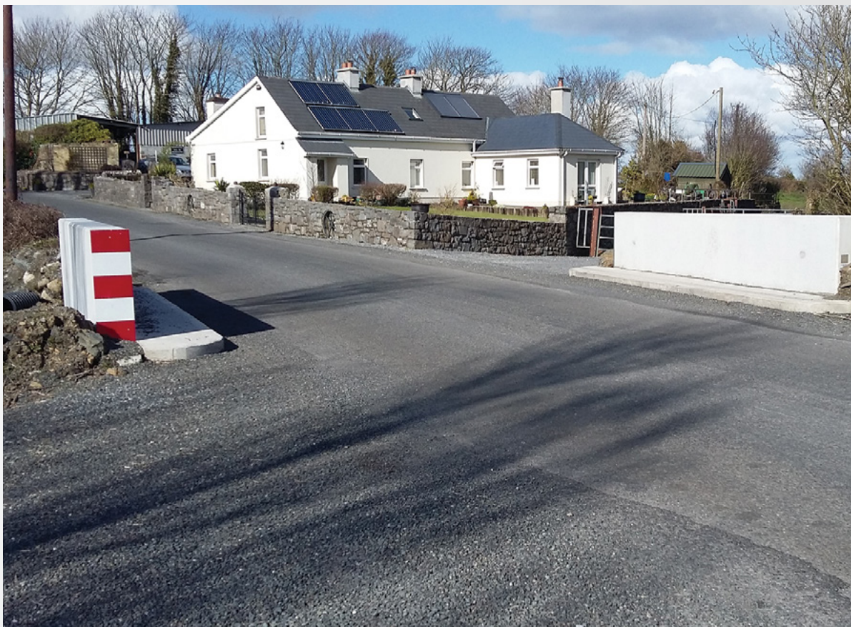
Bridge Improvement Works at Ballyegna.
