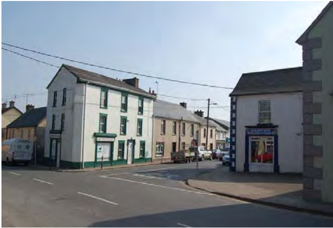
← Figure 10.3: Opportunity Site 2 Photograph of existing junction
