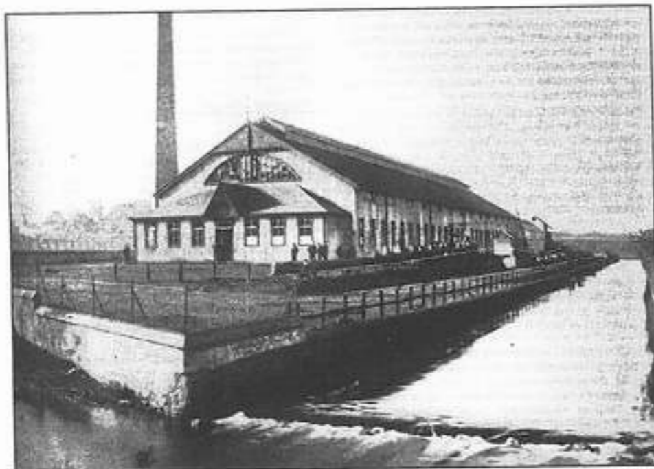
Cleaves Creamery, Tipperary Town, was occupied by workers in 1922 and burnt down during the Civil War.
