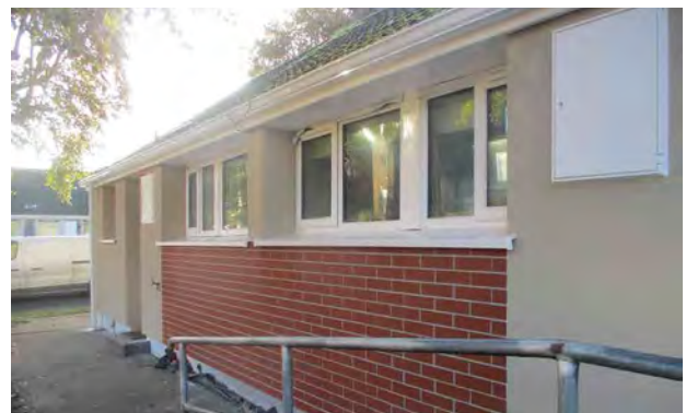
Energy Retrofit 2022 – Schoolhouse Lane, Limerick
