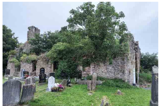
Works at Kilfinnane Burial Ground Before
