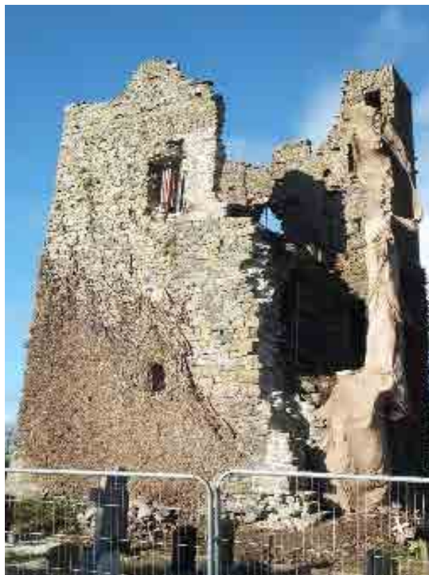
Works at Ballynoe, Bruree After
