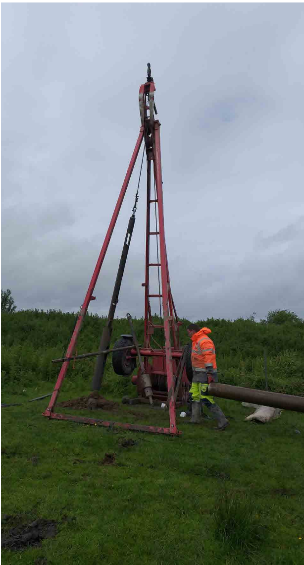
Limerick Flood Relief Scheme - Ground Investigation Works
