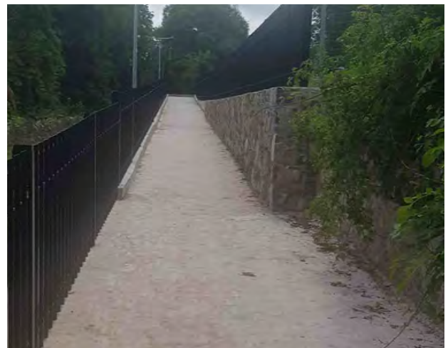
Croom Ramp and Walkway
