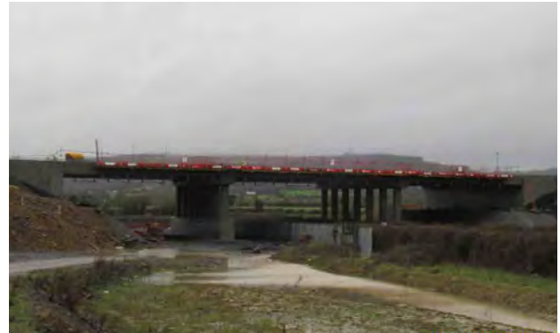
Ballygrennan Bridge under construction
