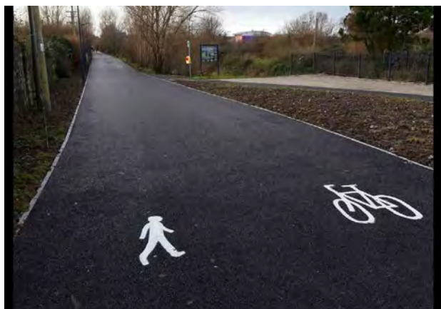
Widened Greenway from Troy’s Lock to Lelia Street along the Canal Bank
