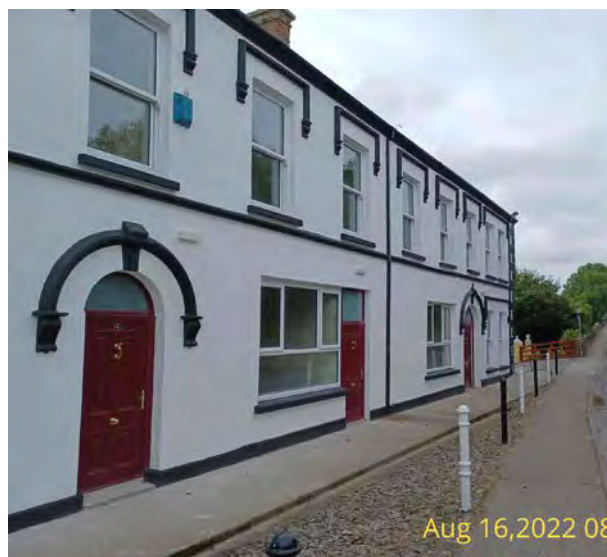
Pallasgreen Property after refurb by owner
