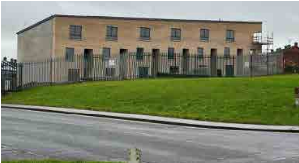
Cliona Park Phase 3 Housing Development Moyross due for completion late Spring 2023
