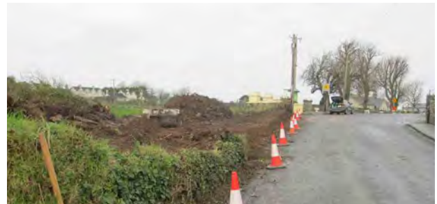
Before – Kiltleely Community Wildlife Area project Town and Village Renewal Scheme 2019
