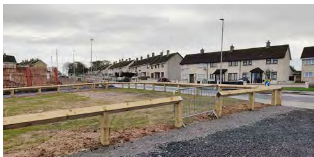
Galvone Arms site Southill post-demolition
