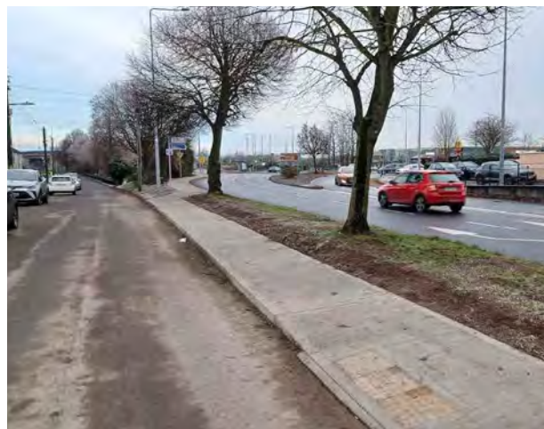
New Footpath Link at Ballykeeffe Roundabout
