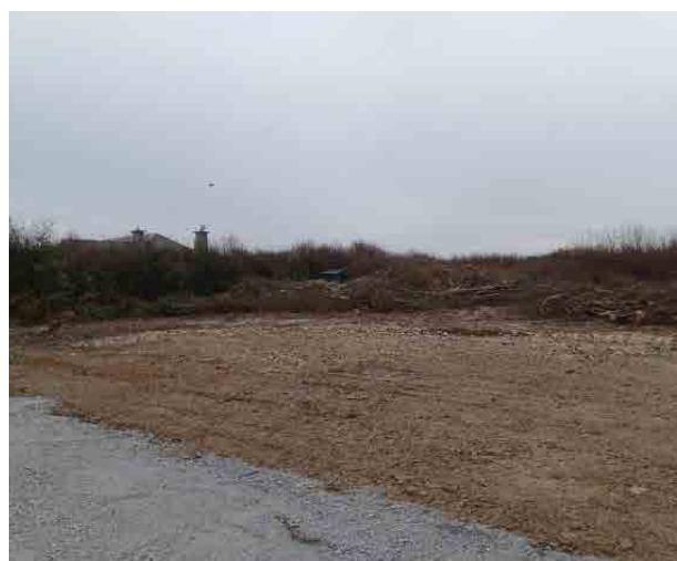
Site Clean Up After
