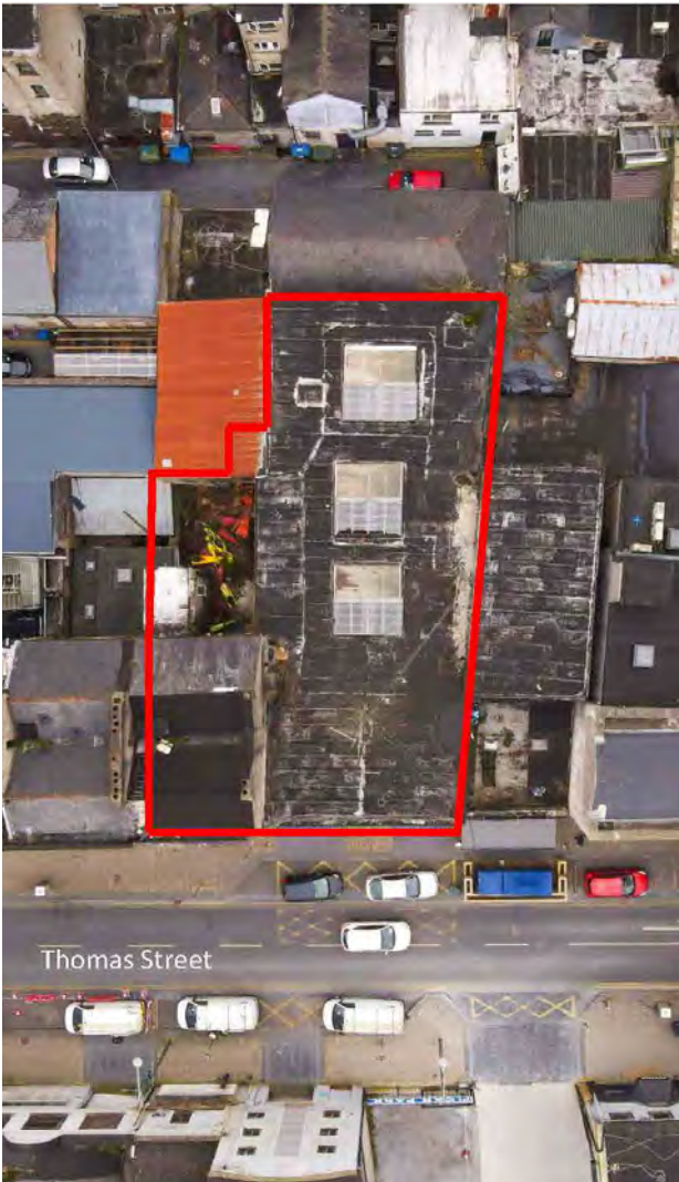
Aerial View of 33 and 34 Thomas Street
