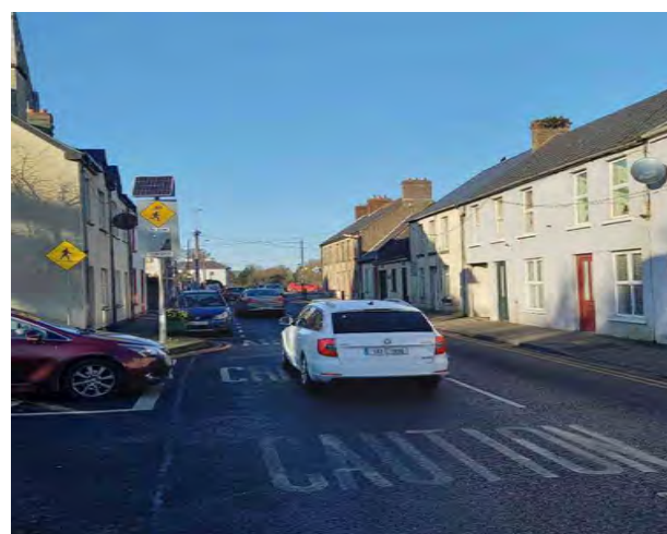
2022 Low Cost Safety Scheme Works Kilmallock Town
