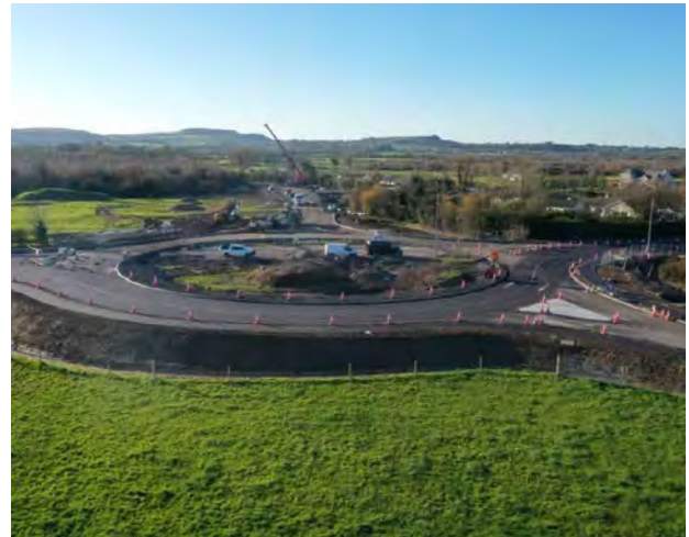
Construction works at N24 Beary's Cross Road Improvement Scheme
