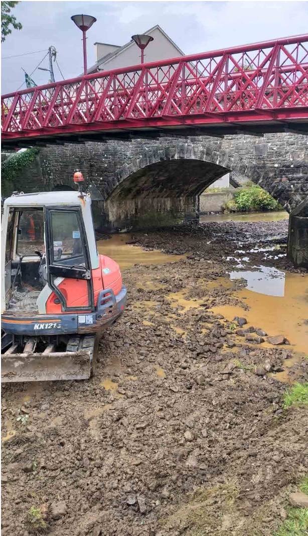
Athea Flood Relief Scheme - Advanced Works
