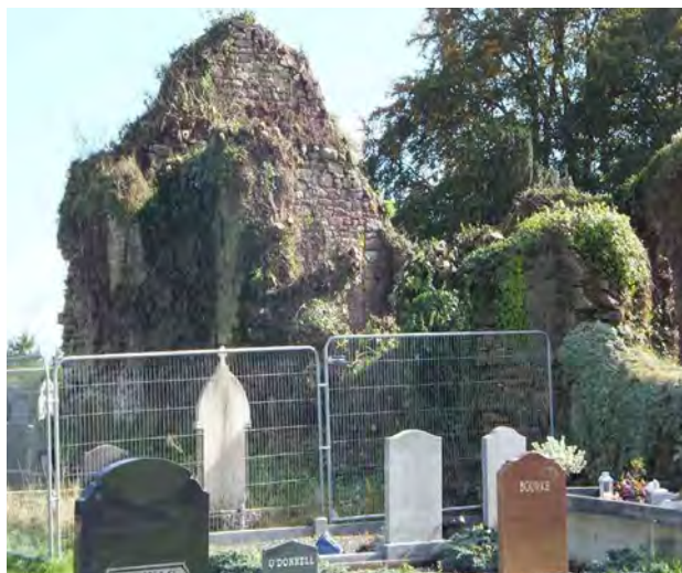
Works at Galbally Church
