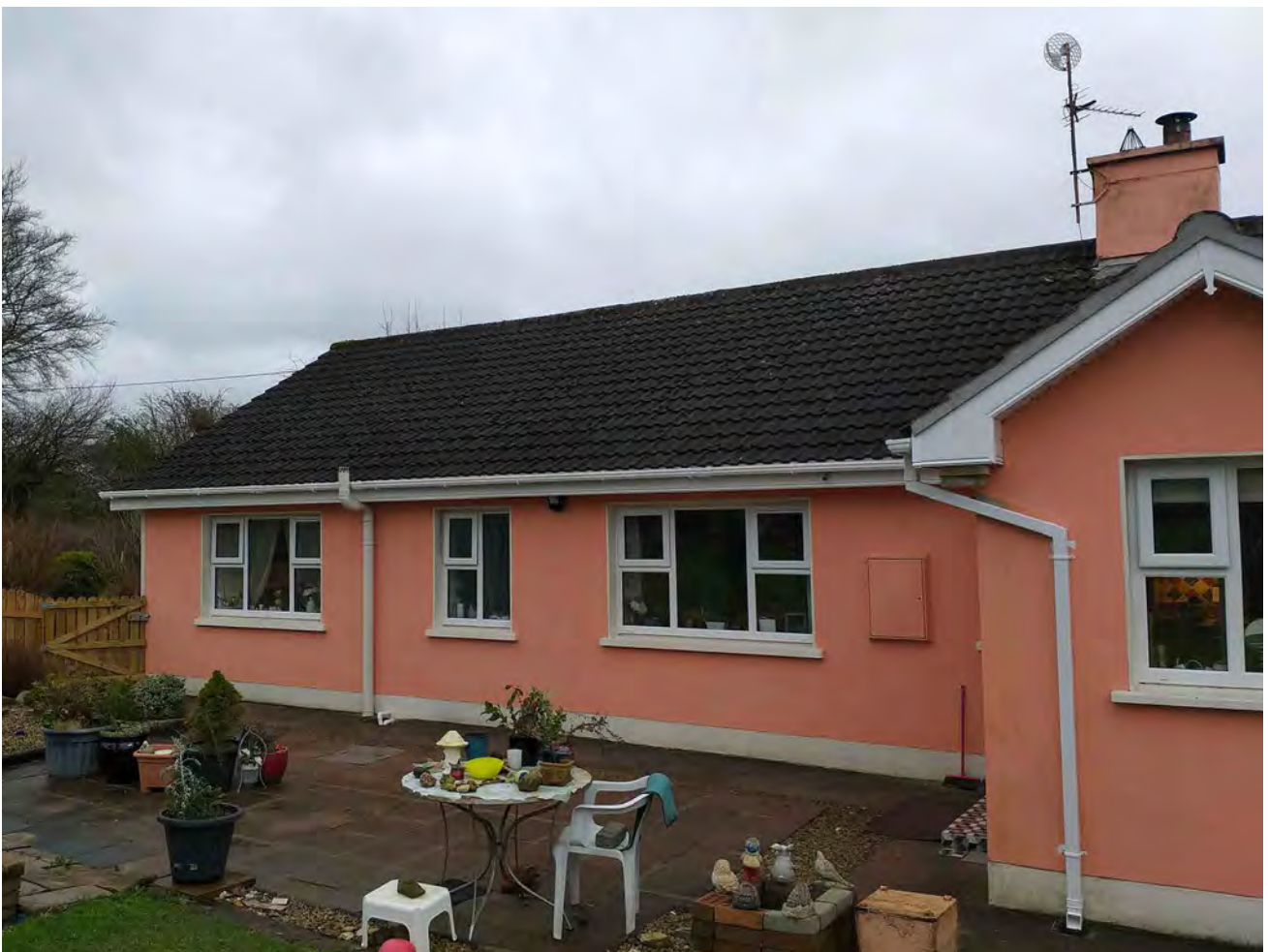
New windows Housing for Older persons grant
