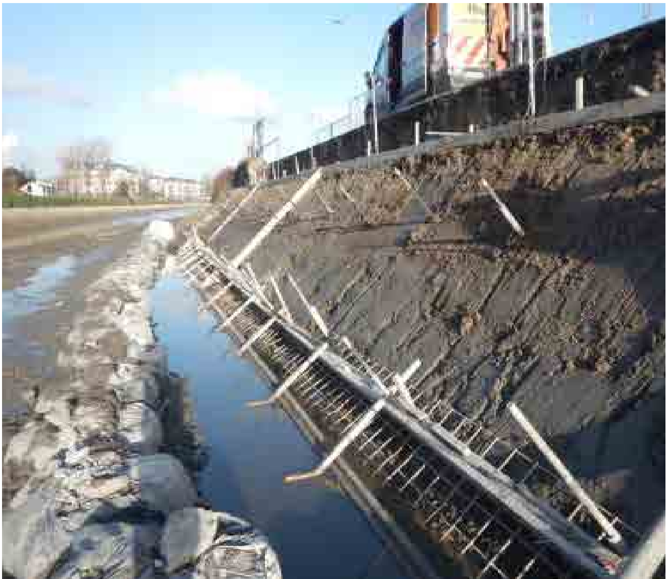
Blennerville Canal Walls - Ground anchors installed, awaiting grouting and masonry finish
