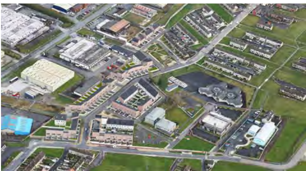
Churchfield Phase 2 Housing Development Southhill due for completion early 2024
