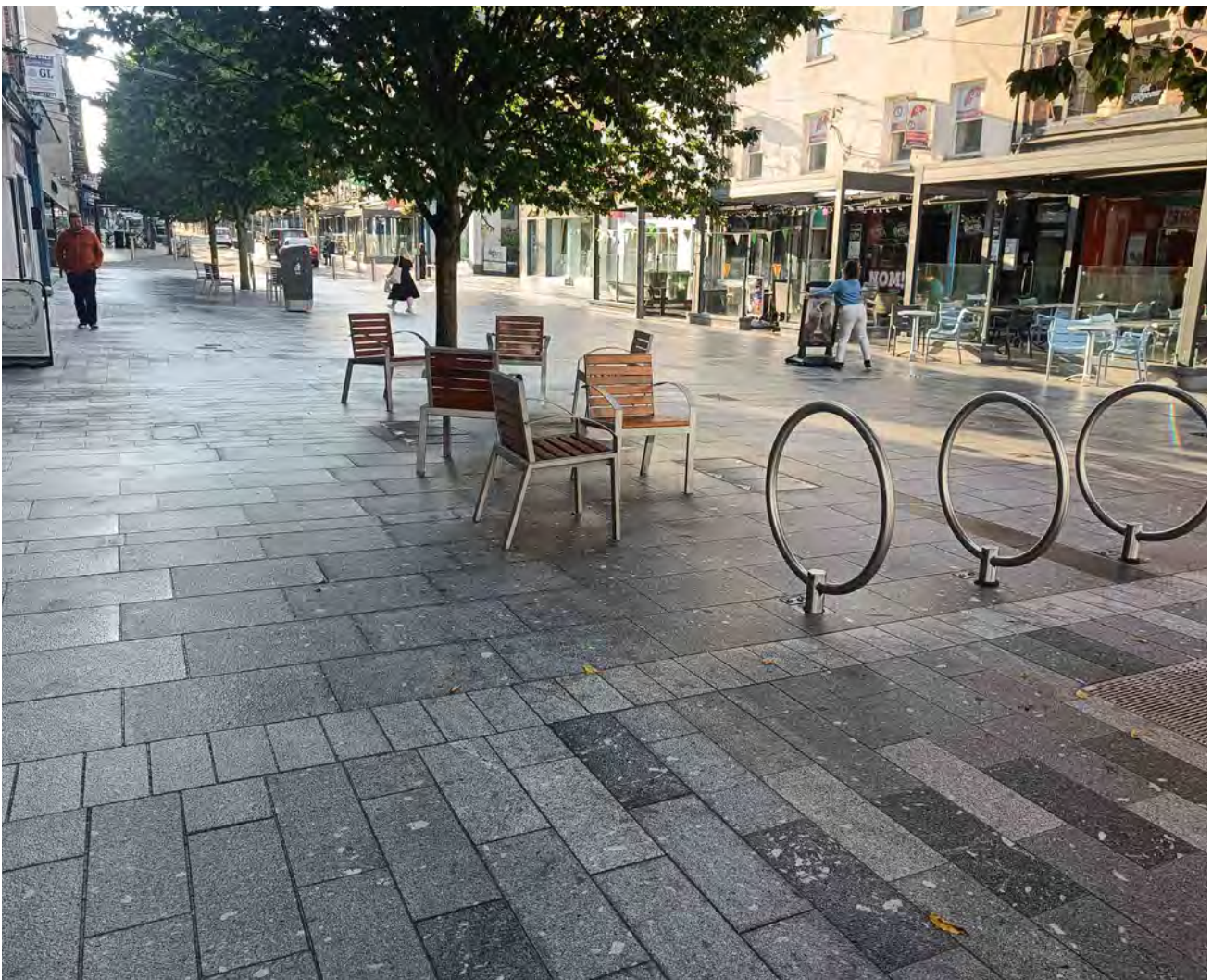
Public Realm Works Thomas Street
