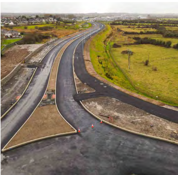
Aerial View of the Coonagh Knockalisheen Distributor Road
