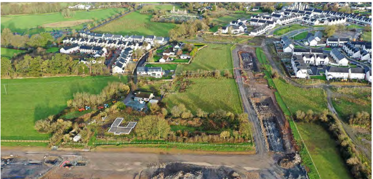
Mungret Link Street - View North to Mungret Gate
