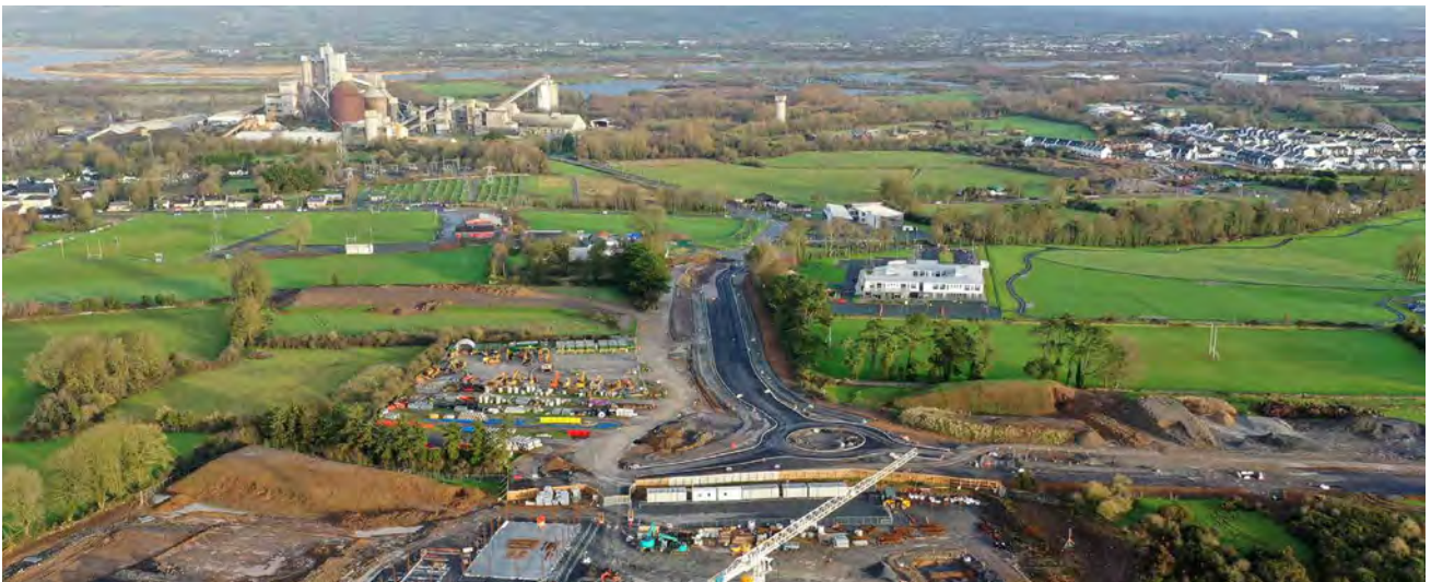
Mungret Link Street - View to North
