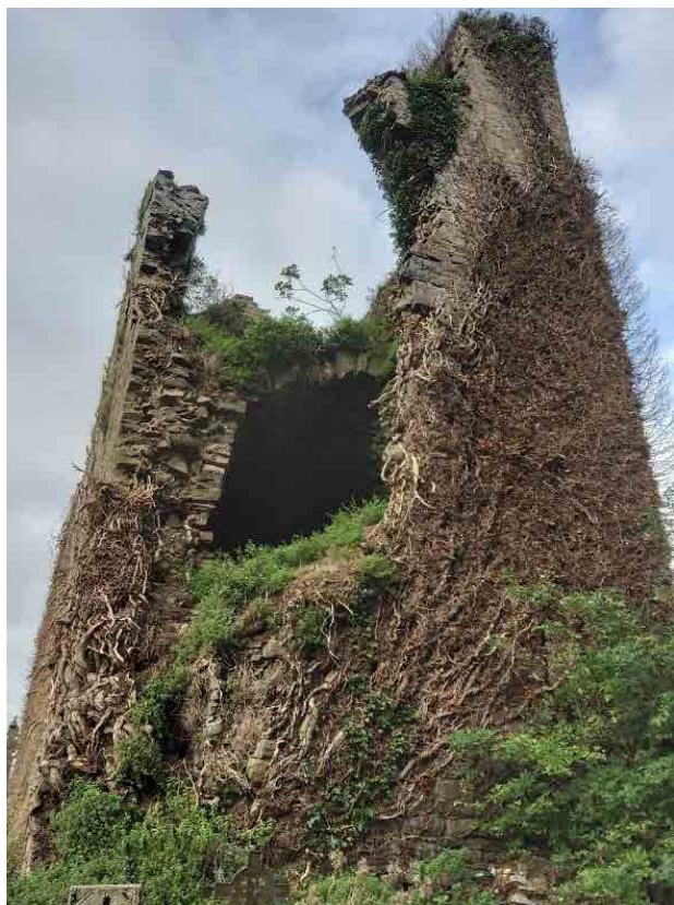
Works at Ballynoe, Bruree Before
