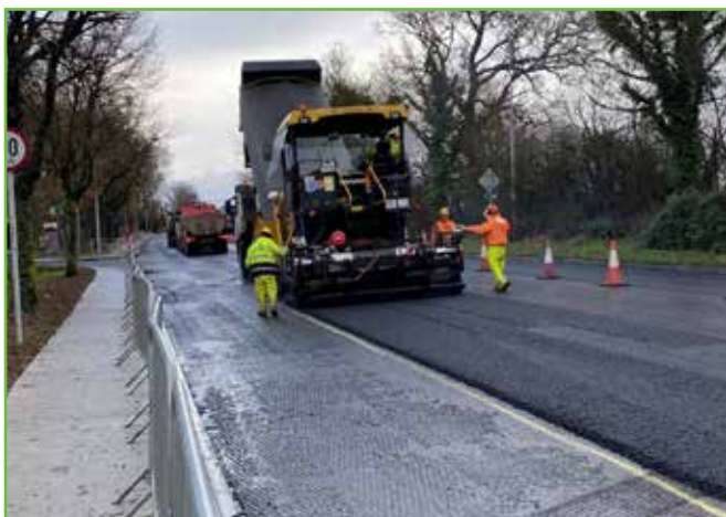
Newcastle West Pavement Works in Progress
