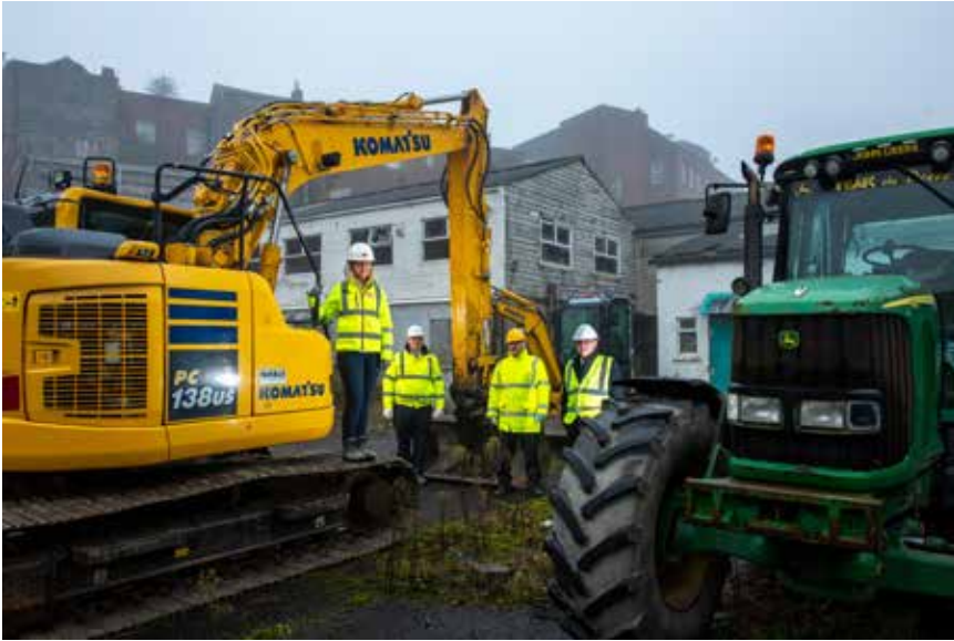
At the commencement of the demolition and enabling works programme at Opera Site by contractor John Sisk & Son Ltd.. Pictured from left: Aoife Munnelly, Site Safety Officer, John Sisk & Son Ltd., David Conway, CEO, Limerick Twenty Thirty, Dr. Pat Daly, Chief Executive, Limerick City and County Council, Mayor of the City and County of Limerick, Councillor Michael Collins.
