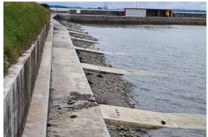
New slipway at Glin Pier
