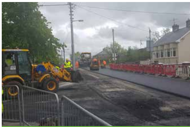
Mcadam overlay works at Bishop Street, Newcastle West
