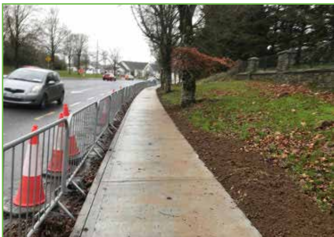
Footpath Works as part of Newcastle West Pavement Improvement Scheme
