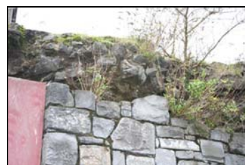
Plate 3.135. Facing stone and core masonry
