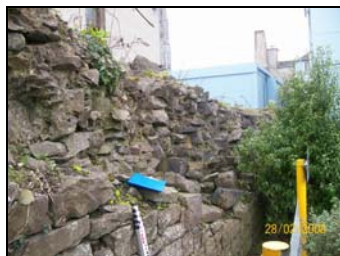
Plate 3.108. Core exposed
