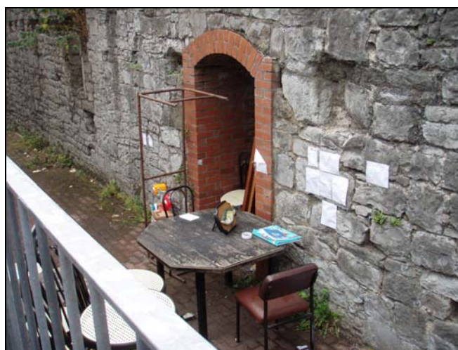
Plate 3.128 Restored ope in external face of stretch, from southwest
