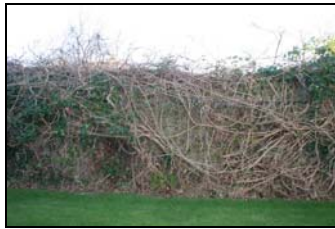
Plate 3.41. Extensive woody plant growth on section 2
