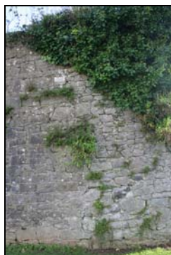
Plate 3.22a. Transition between tower and wall facing stones
