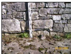
Plate 3.90. DPM showing change from original modern facing stone
