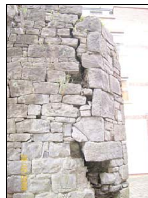
Plate 3.159. Structured crack in gate opening
