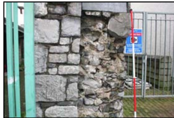
Plate 3.138. North end showing modern and original masonry
