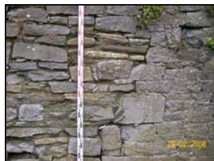
Plate 3.109. Change of masonry: medieval to 19 th century
