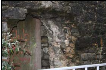
Plate 3.140. Detail of masonry core in opening
