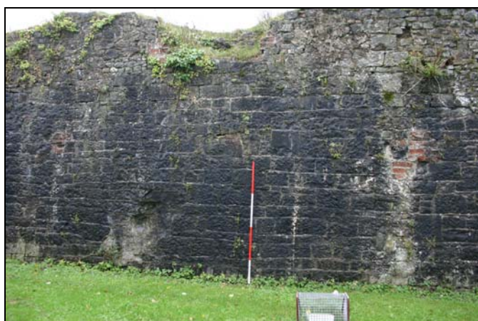
Plate 3.49. View of southern section of stretch, note dressed stone and possible later insertion of a large window at top of wall
