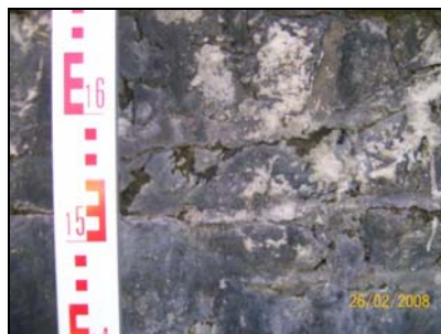
Plate 3.58. Detail of modern pointing
