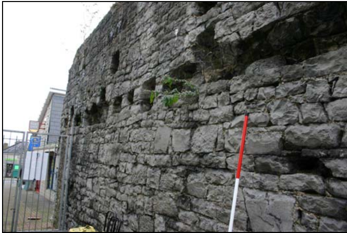
Plate 3.130. External face of City Wall, with joist holes inserted, from southwest
