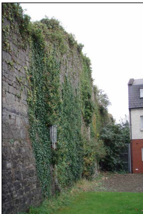
Plate 3.88. External face of City Wall at southern end, note slight batter and ROW
