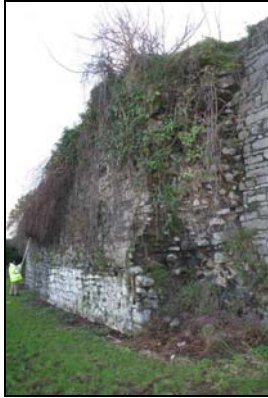
Plate 3.38. First part of section 1 showing exposed core masonry
