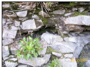
Plate 3.61. Core masonry
