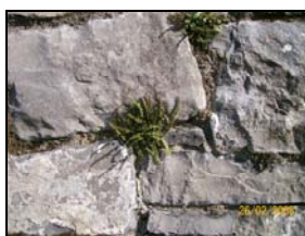
Plate 3.91. Non wood plants on facing stone
