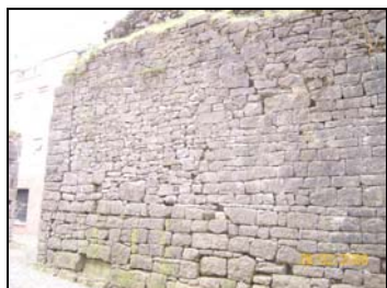
Plate 3.160. Original facing stone and later repairs
