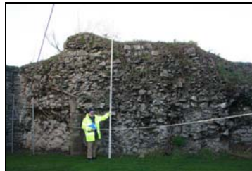
Plate 3.36. Exposed core masonry in section 1.
