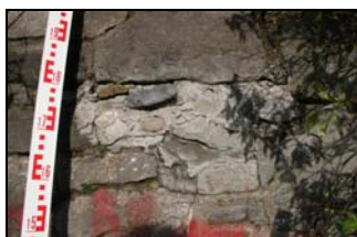
Plate 3.18.Cementitious repair on tower
