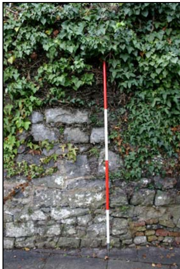
Plate 3.44. View of fabric of medieval City Wall, from west. Note infilling at base
