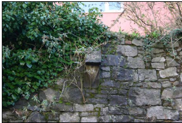
Plate 3.145. Single corbel on external face
