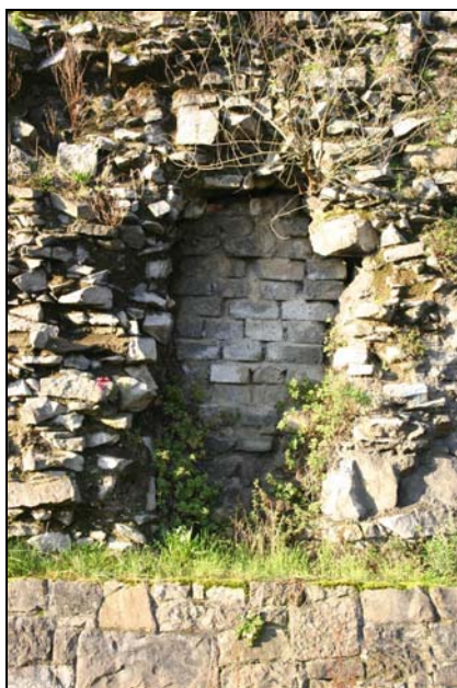
Plate 3.81. Breach, modern infill and rubble core exposed, external face of City Wall
