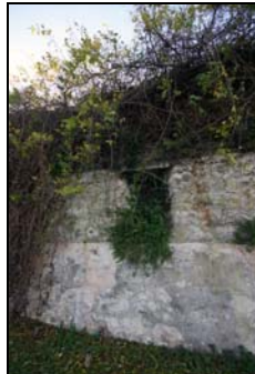
Plate 3.35. White wash render to exterior of wall
