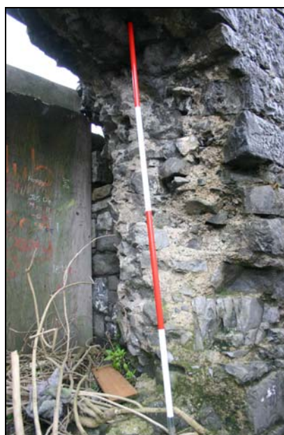
Plate 3.129. Original rubble core from northwest
