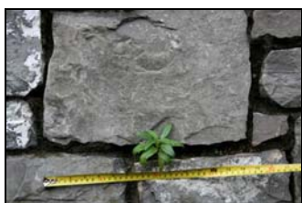
Plate 3.136. Detail of modern facing stone
