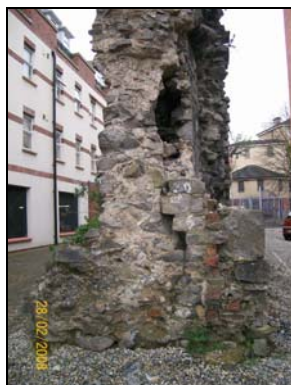
Plate 3.157. Structural Collapse at northern end
