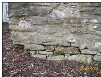
Plate 3.120. Wall base eroded
