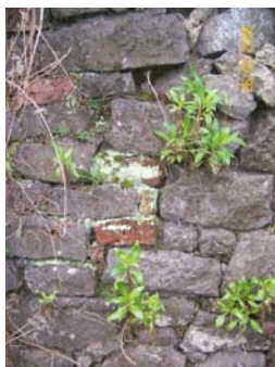
Plate 3.53. Evidence of pre 20 th century repairs.
