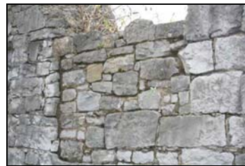
Plate 3.141. Opening filled in with masonry
