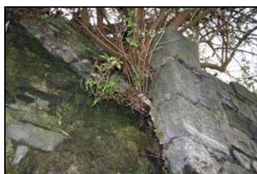
Plate 2.133 Detail of vegetation damage
