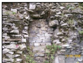
Plate 3.93. Concrete block repair.
