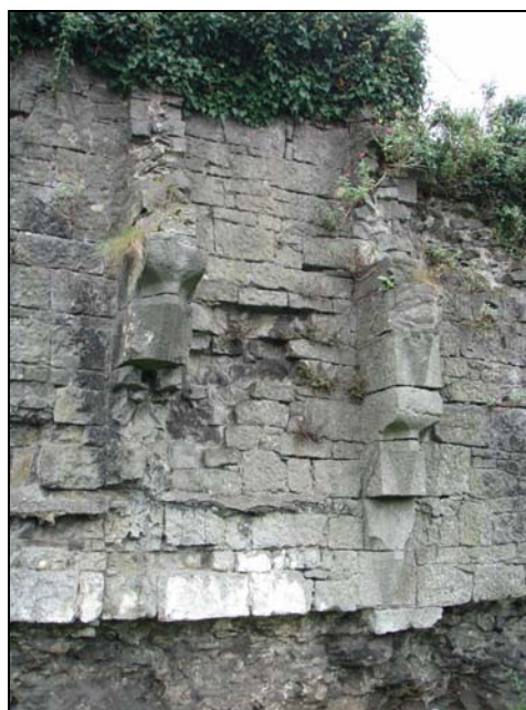
Plate 3.48. Detail of corbelled structure
