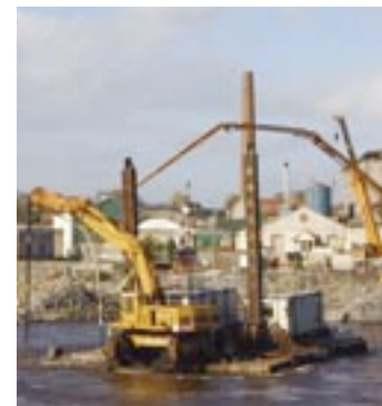
LIMERICK MAIN DRAINAGE_
